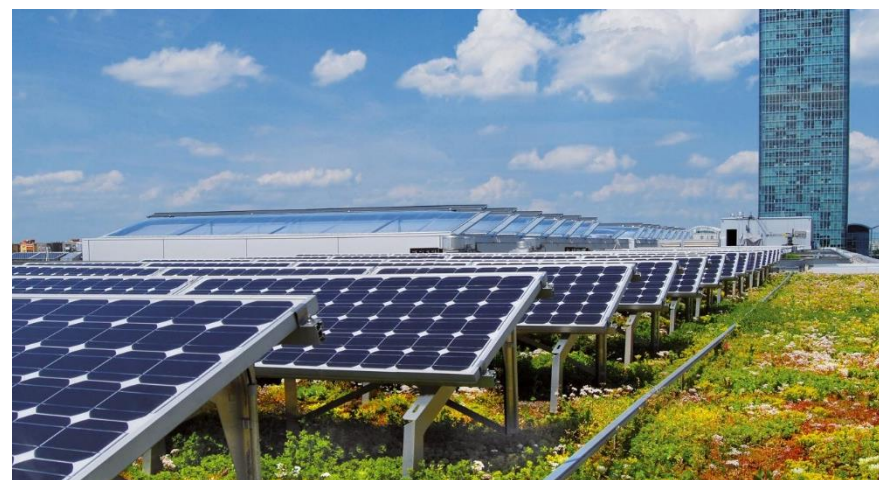
Figuur 56 The Munich Technology Centre, München. Bron: ZinCo Green Roof Systems
