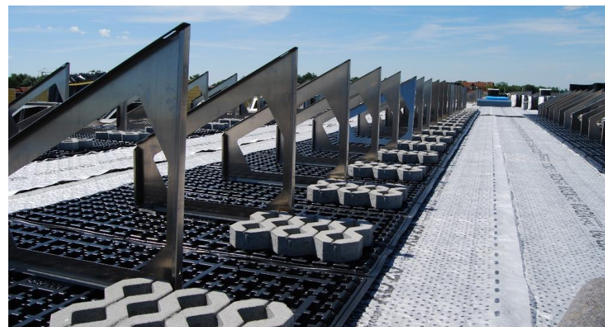
Figuur 57 The Munich Technology Centre, München. Bron: ZinCo Green Roof Systems
