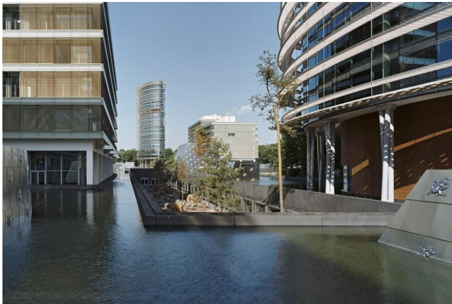
Figuur 16 Open permanent waterdak. Walterboscomplex. Apeldoorn. Nederland. Bron: Neutelings-Riedijk Architects
